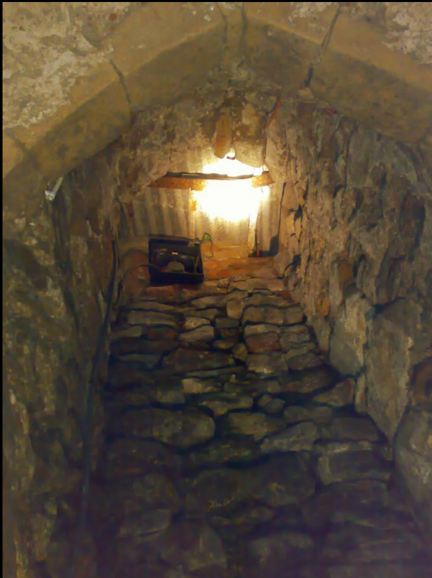
BELOW: Bricked up or removed window / light well: About two thirds of the vaults would have had windows set into the front wall (occasionally a side wall if it was on a corner plot) and they would have had very steep sills as seen in the picture below. A lot of the vaults would have just relied on natural light from the doorway to illuminate them. This was alright when the vault was a single room, but in the case of the 3rd vault we saw, the light quickly faded after the first room and was virtually non-existent by the third room in, which would have made them quite spooky.
