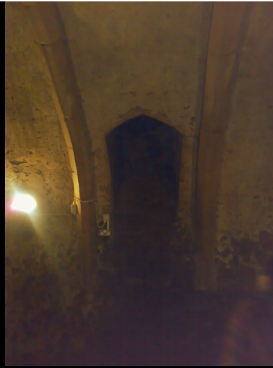
BELOW: Bricked up or removed window / light well: About two thirds of the vaults would have had windows set into the front wall (occasionally a side wall if it was on a corner plot) and they would have had very steep sills as seen in the picture below. A lot of the vaults would have just relied on natural light from the doorway to illuminate them. This was alright when the vault was a single room, but in the case of the 3rd vault we saw, the light quickly faded after the first room and was virtually non-existent by the third room in, which would have made them quite spooky.
