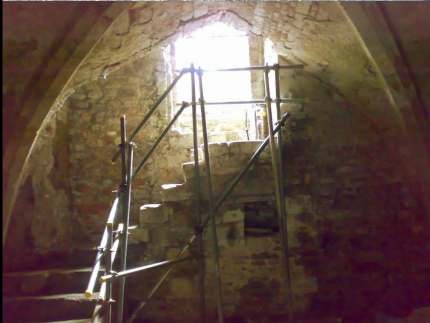
BELOW: This vault differs from the previous 2 as it has more classical (and more commonly seen) diagonal ribs, whereas the others are barrel-vaulted, ie: the ribs are purely between the sides crossing the floor area at 90 degrees.
