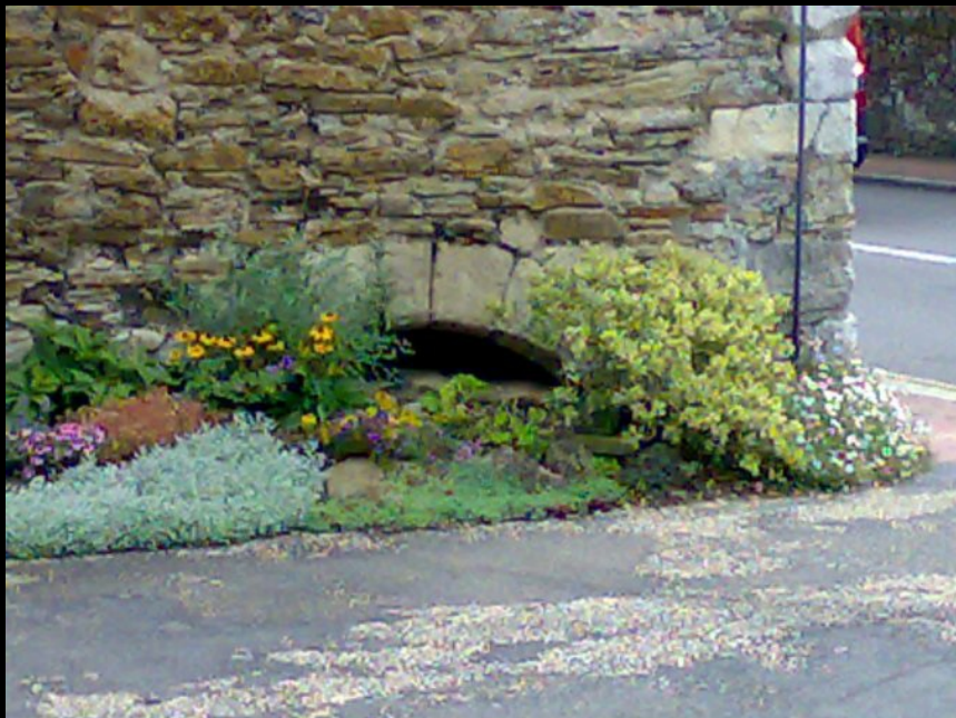
ABOVE & BELOW: Everywhere we looked there was evidence of more vaults, whether unused or intentionally blocked off. The Heads (or tops of the visible entrances) to the vaults appear above street level in the lower facade of the building above it. Suggestions that the street level was a lot lower at the time of construction than it is today can be discounted, as the visible access to the vaults has remained the same.
