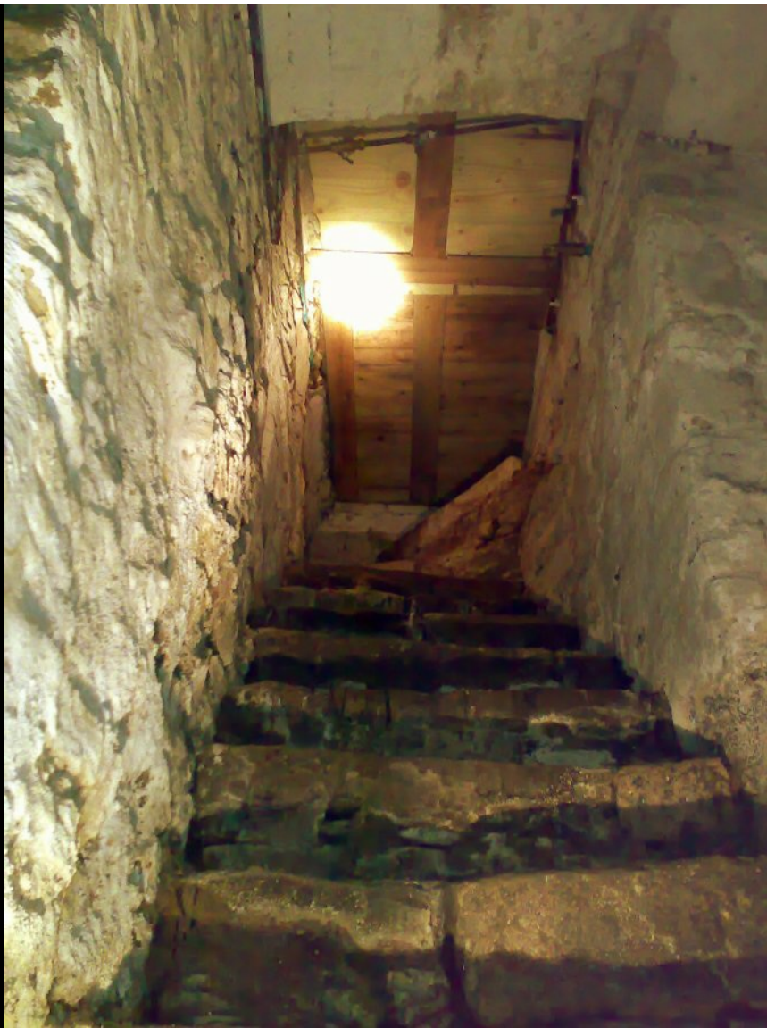
BELOW: In most cases there would have been double wooden doors set into the entrance arch. Originally these would have opened into the vault and would have required quite a lot of room to open fully. This meant that the ground floor of the building above the doorway of the vault would have been raised above the rest of the floor area, resulting in a sort of step along the outer wall of the room. In a lot of cases, the hatches seen at street level in the present day are later additions. It is thought that, originally, there would have been porch-like structures built over the vault entrances to shield them from bad weather.
