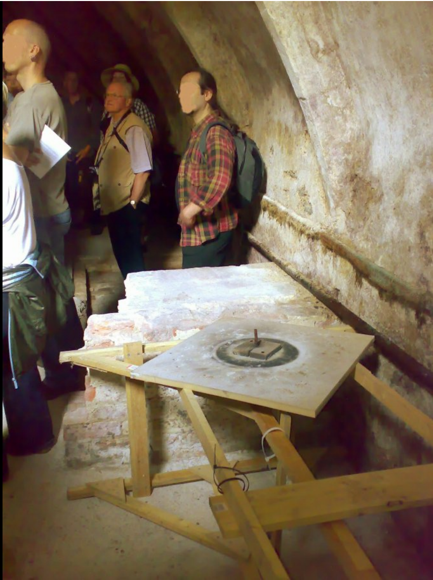
BELOW: Eight of the vaults which survive into the present day have a second smaller staircase leading to the house above. In some instances, the staircase to the rear lead up to a rear courtyard. There are 3 such examples in the town.
