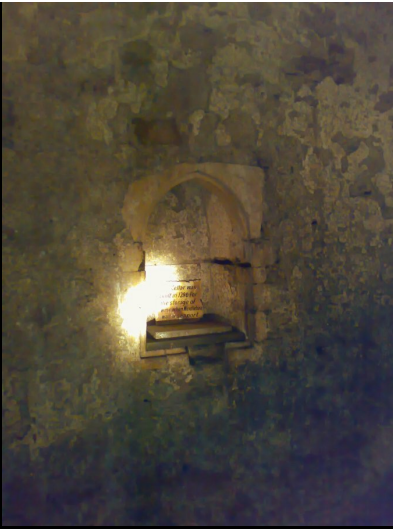
BELOW: Bricked up or removed window / light well: About two thirds of the vaults would have had windows set into the front wall (occasionally a side wall if it was on a corner plot) and they would have had very steep sills as seen in the picture below. A lot of the vaults would have just relied on natural light from the doorway to illuminate them. This was alright when the vault was a single room, but in the case of the 3rd vault we saw, the light quickly faded after the first room and was virtually non-existent by the third room in, which would have made them quite spooky.
