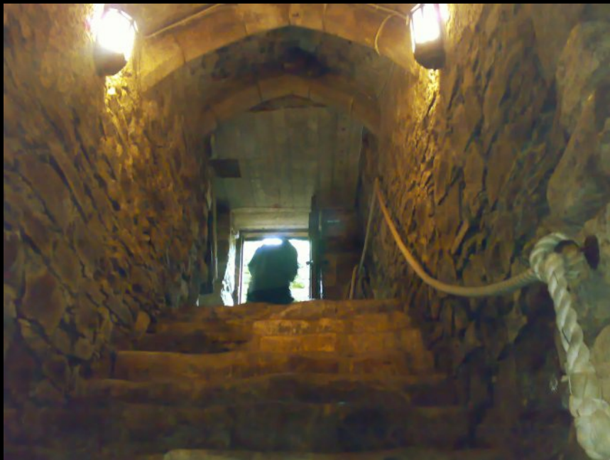
BELOW: The floors of the vaults were usually made of compacted earth or slabs of Tilgate Stone, as in the construction of the walls. In some vaults, the floor has been dug out to the level where the stone is naturally occurent as strata (ie: there already - very lazy!)
