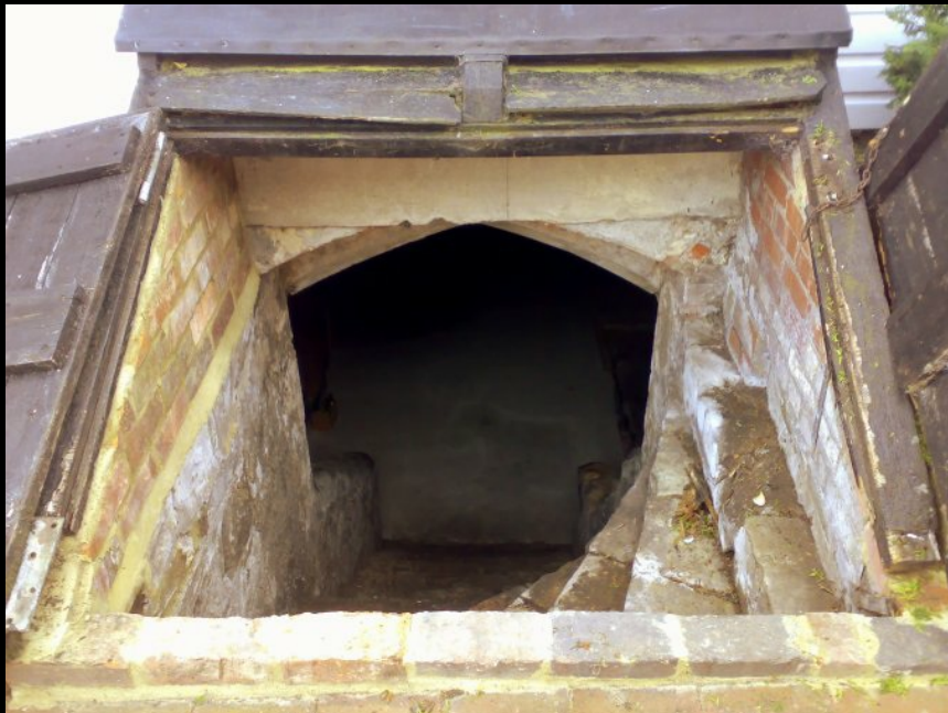
BELOW: In most cases there would have been double wooden doors set into the entrance arch. Originally these would have opened into the vault and would have required quite a lot of room to open fully. This meant that the ground floor of the building above the doorway of the vault would have been raised above the rest of the floor area, resulting in a sort of step along the outer wall of the room. In a lot of cases, the hatches seen at street level in the present day are later additions. It is thought that, originally, there would have been porch-like structures built over the vault entrances to shield them from bad weather.
