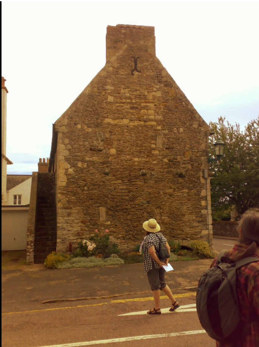
ABOVE: As I've mentioned elsewhere in this part of the website, Winchelsea was a mass of architectural contradictions and this building was no exception. It is a mass of blocked up windows and doorways, all in stone of course. There were so many different types and sizes of stone used, sometimes rendered also, that the place looked like a huge patchwork quilt. As the requirements of the building have changed, the walls are as readable as a notebook. Incredible.
