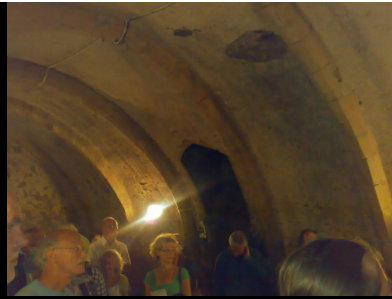
TOP- LEFT & RIGHT: The walls of the vaults are built up from slabs of Tilgate Stone which is laid in rough courses. The faced surface is just a rough cement render apart from those withing vaults with windows, where the walls were quite highly decorated.
