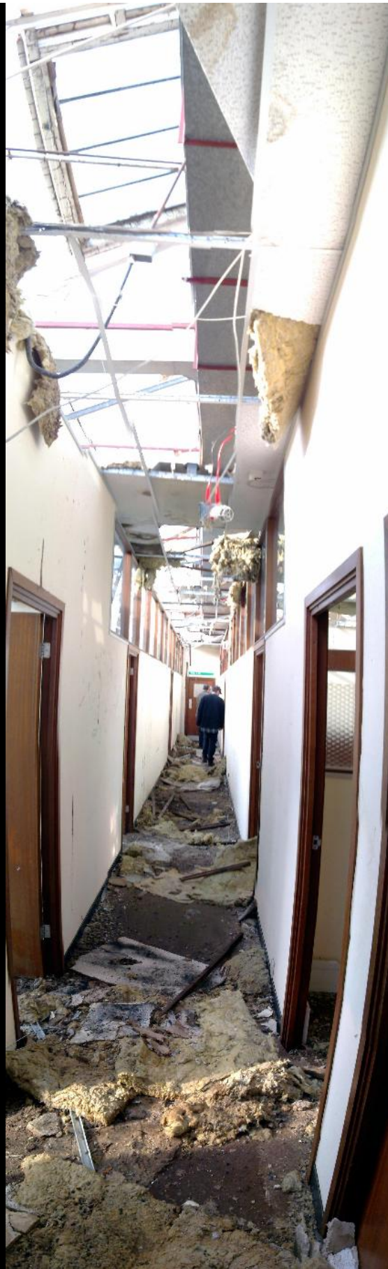
ABOVE: If you want to give your position away to security really easily, go where there are loads of pigeons. There were loads of the little buggers in here, plus the demolition team had crunched the roof off, so we took our time through here and tried not to dislodge too many.
