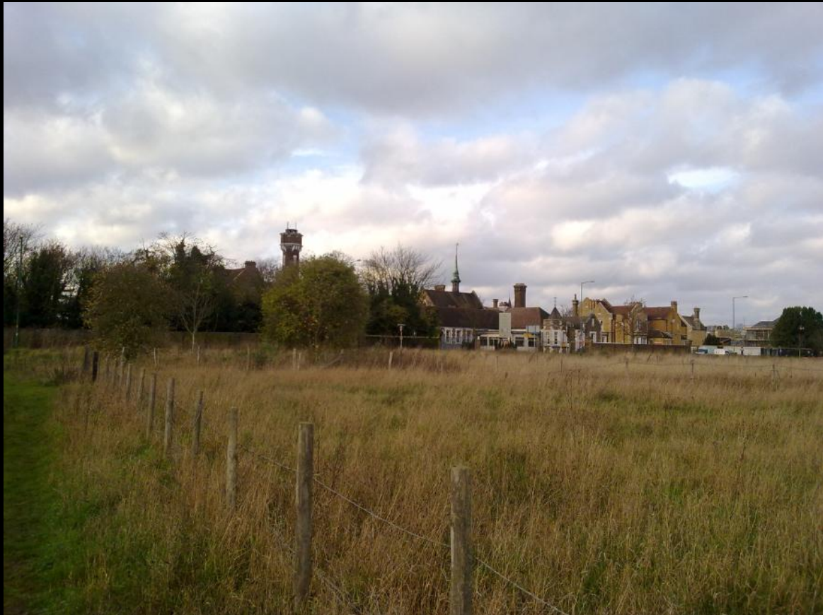
BELOW: With the outer perimeter wall out of the way, the whole glorious panorama of the Stonehouse Asylum spread out before us. It is an incredible looking place. We did wonder if the security fence went all the way round the site. It does, but it also abutts the perimeter wall at one point, and we were luckily able to find it without too much difficulty, as I've mentioned previously, hats off to the security bods: this place was nigh on impenetrable, which explains why it's in such great condition. Look at the security at Hellingly over the last decade and the state of the place. There's just no comparison, really - Hellingly got trashed as just about anyone could just walk into it until it was far too late.
