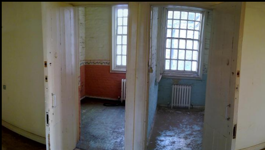
ABOVE & BELOW: We were a little baffled by these two rooms: firstly - were the residents given the choice of deciding the colour of their rooms? The other thing that we couldn't figure out was the presence of huge amounts of Copper Oxide in this room. It is clearly quite a recent thing as it's clearly happened after the placement of the chairs. We did wonder whether the proximity to the room with all the murals had some kind of significance - possibly art materials? Copper Oxide is used extensively in pottery, but there is nothing in the way of pottery related paraphenalia to support this hypothesis...
