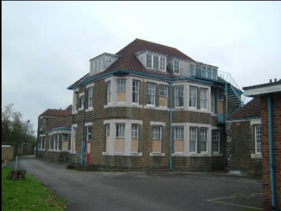
BELOW: So... the boiler room was a non-starter. Next we thought about high up things that most people wouldn't see and the security guards would hopefully not want to risk their necks checking out, like all these mad UrbEx freaks. Hmm... fire escapes usually have doors leading onto them!
