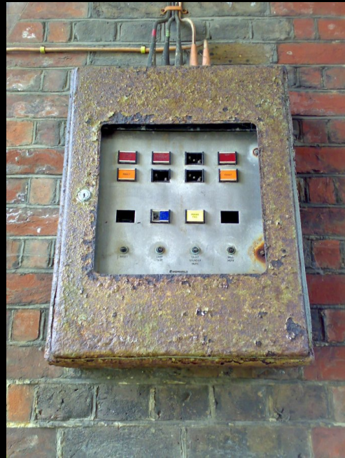
At the southern end of the accomodation block is a gateway, which appeared to be the main way into the site at one time. The gate was automatically controlled and the switchgear is shown BELOW.
