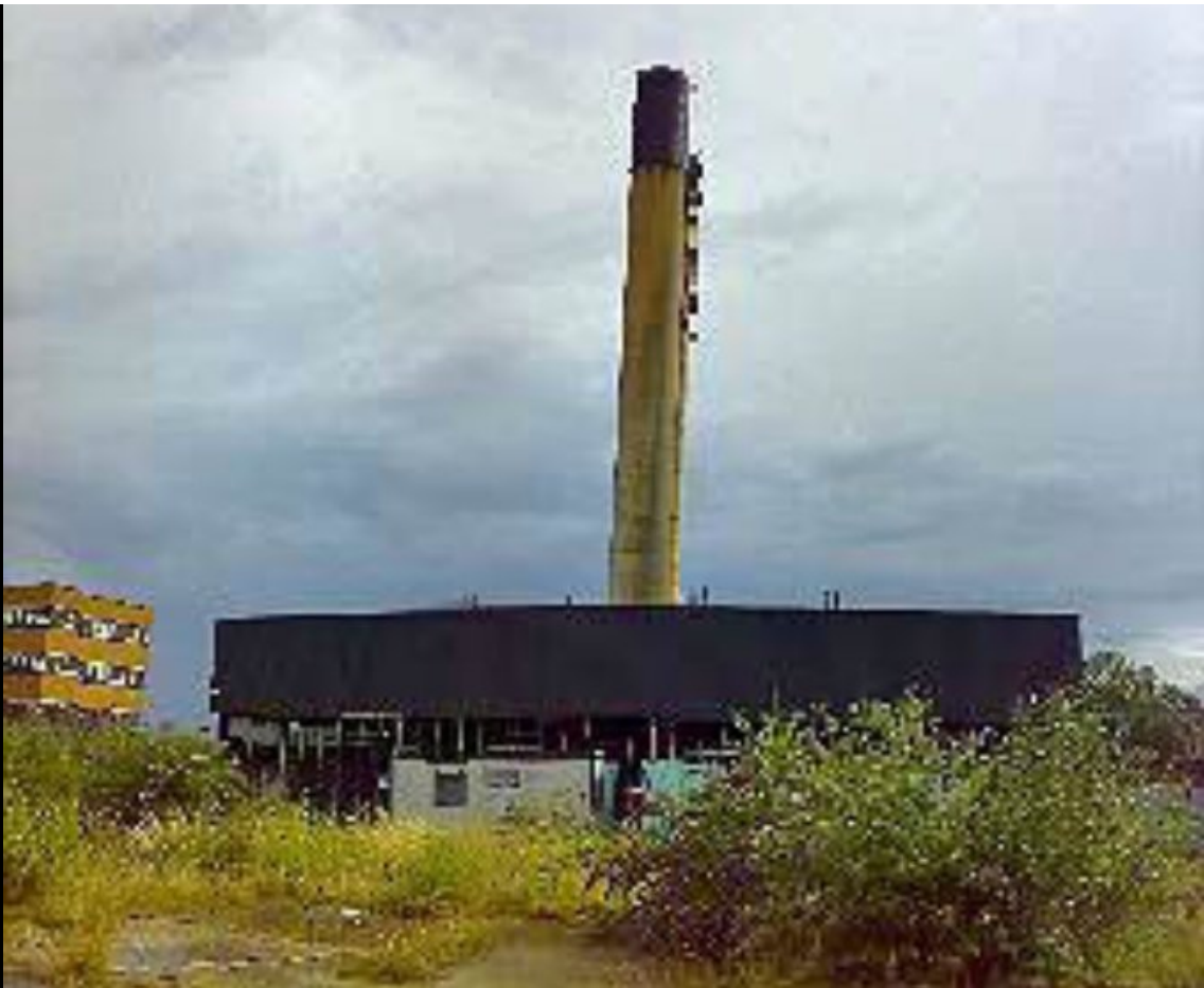
ABOVE: This is what most people look for when they go to Southlands, it seems to certainly be what most people remember most about the place. But the heating plant beneath it is derelict and on the part of the site that we were heading for.
