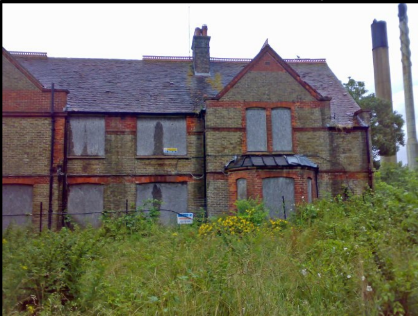
BELOW: Parting shot of the block with the Hall, Kitchens and Canteen Hall, looking back due South.
