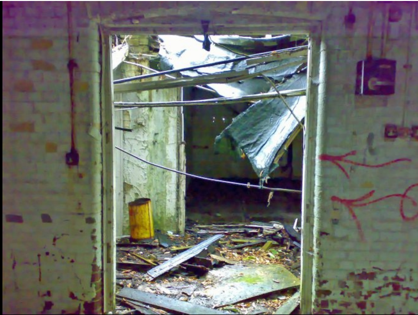
BELOW & BELOW: A lot of the rooves around the Dining Hall and Kitchens were heavily water damaged and had either fallen in or were in the process of falling in. We proceeded with care.
