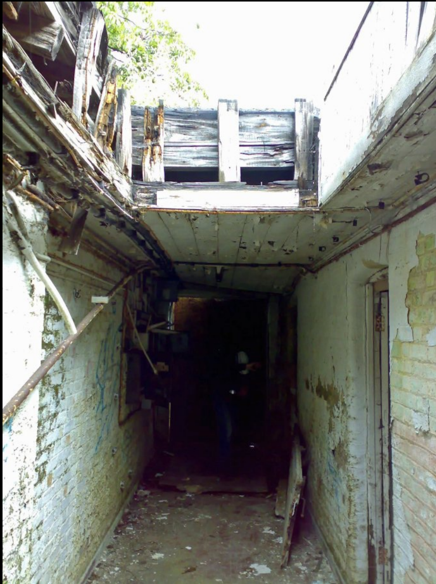
BELOW & BELOW: A lot of the rooves around the Dining Hall and Kitchens were heavily water damaged and had either fallen in or were in the process of falling in. We proceeded with care.
