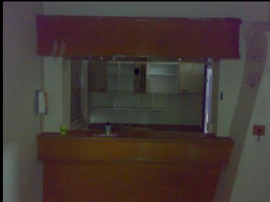
ABOVE: The hospital is literally littered with these little reception style hatches! We are guessing for signing into or out of a certain department or ward? There was not much space round the back to contain drugs so we don't think this was a dispensary.
