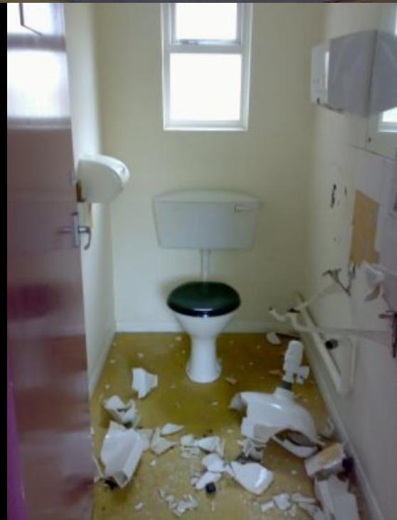
ABOVE: Sadly, it appears our friend "Sink Smashing Man" had got here before us. You may remember from the other trek pages that there wasn't a single sink we could find left intact at either Hellingly or Southlands Hospital! We have yet to understand the attraction...
