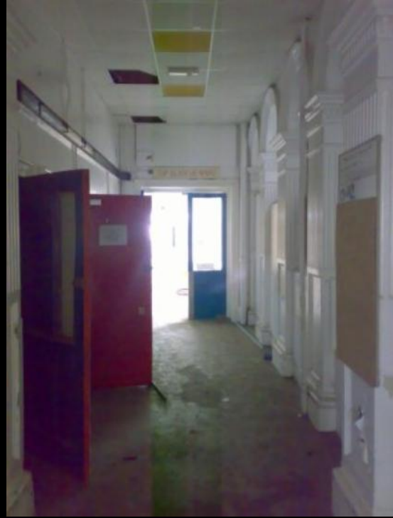
ABOVE: As I have mentioned previously, a lot of the original Victorian arches are hidden behind plaster board on the lower floors. Thankfully, here they have been left alone and they look wonderful. This is just outside the doorway to The Blanche Ward.
