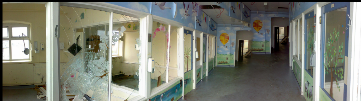
BELOW: Wards on top floor, a strange fusion of very pretty murals and harshly broken glass.
