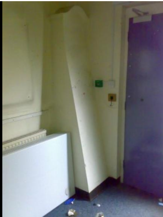
ABOVE: This was quite interesting when we found it: there were 2 of these (I suppose we should call them) buttresses, one on either side of a doorway. This was a very Victorian feature and was used extensively to strengthen tall walls - there are 2 further stories above. It also nicely illustrates the way the site has been extended as it has outgrown the original buildings so that some originally external features appear a little incongruous inside.
