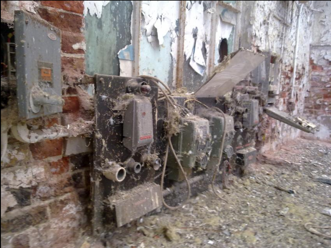
BELOW: Same workshop looking in the opposite direction towards the foreman's office.
