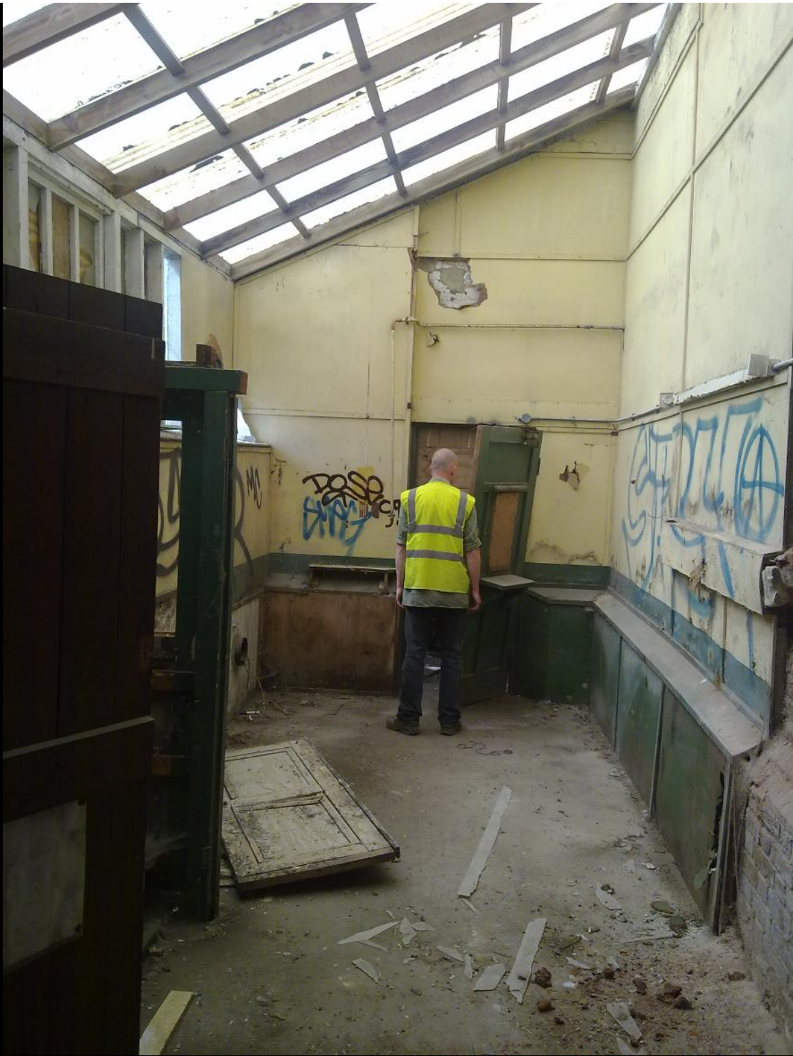
BELOW: More lovely electrical switchgear.
