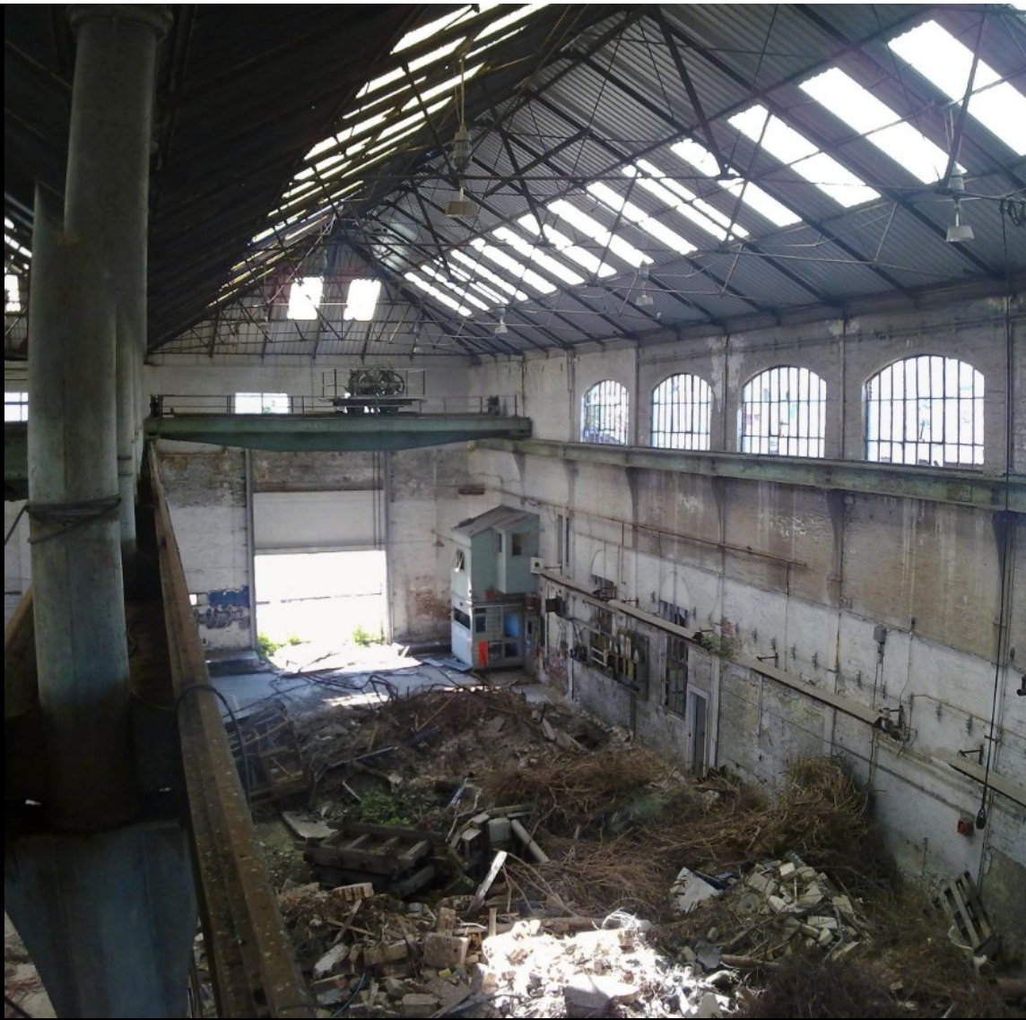
BELOW: We found this smaller workshop just off the main ones, to the south. Note the fantastic array of electrical switchgear and the decades of pigeon crap. There is evidence that there may have been overhead line shafts in this workshop: the walls bore signs of being repaired where fixing plates would have been attached to support the line shaft fixings.
