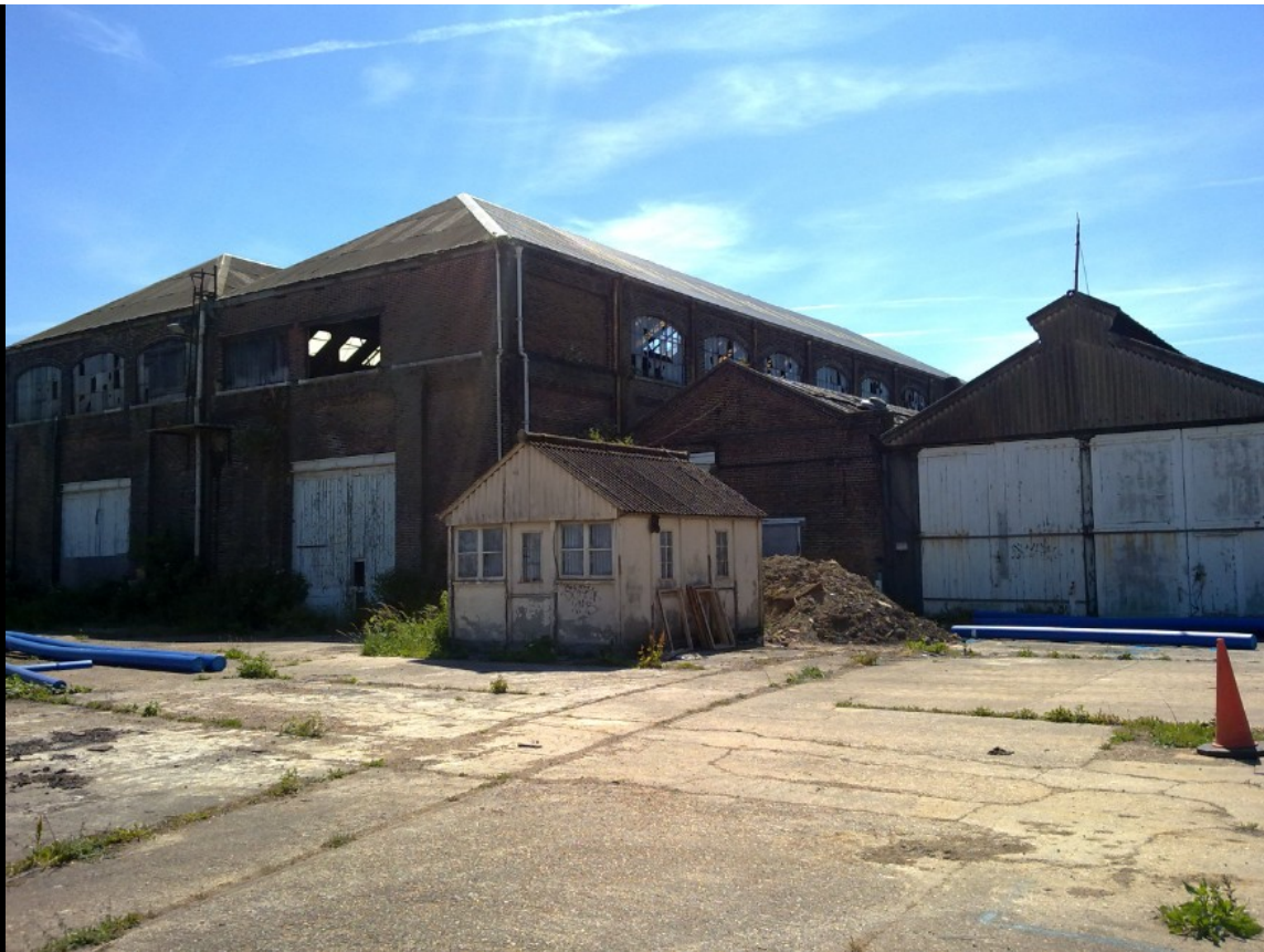
ABOVE: Here we are on the wrong side of the fences... The site is pretty much wide open, so any supposed workmen could come and go pretty much as they pleased - hence the use of PPE as camouflage. It does look as though the site is going to be redeveloped soonish, as there was a mini digger on site and a few bits and bobs of pipework.
