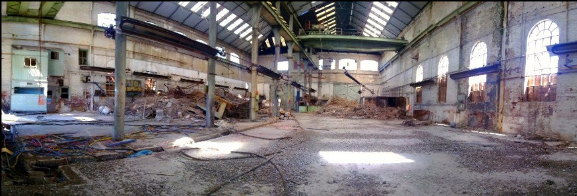
BELOW: This vertical panoramic shot gives a better impression of the scale of the place - it is quite a large building. It also shows one of the overhead gantry cranes in better detail - they are hand operated and (if you were brave enough to venture up onto the walkway between the pillars), it is still just about possible to move them around. Someone has recently used one to hook a length of the heating and lighting strip.
