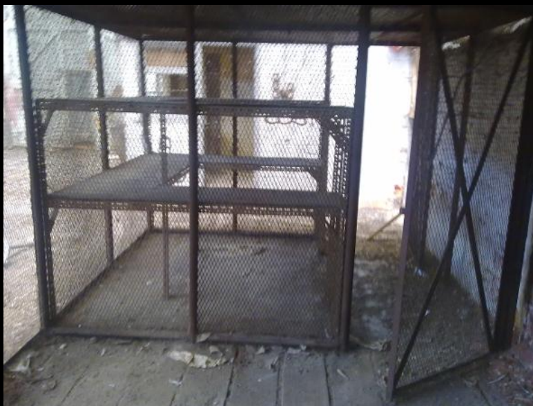
ABOVE & BELOW: Metal store and nut & bolt / fixings stores in the next block along.
