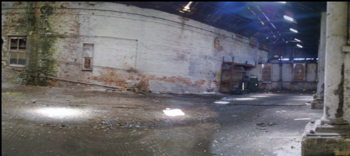
BELOW: Remains of a workshop area just off the main open area, at the rear of the building.
