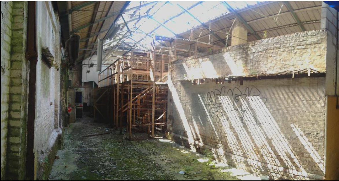
BELOW: The nut&bolt and fixings stores are something to behold. It must have taken several people quite a long time to construct this structure, as it is made entirely from pre-drilled angle iron. We aren't sure what sort of area this area covers, but it is sufficiently strong that walkways have been constructed over the top of it. Very impressive!
