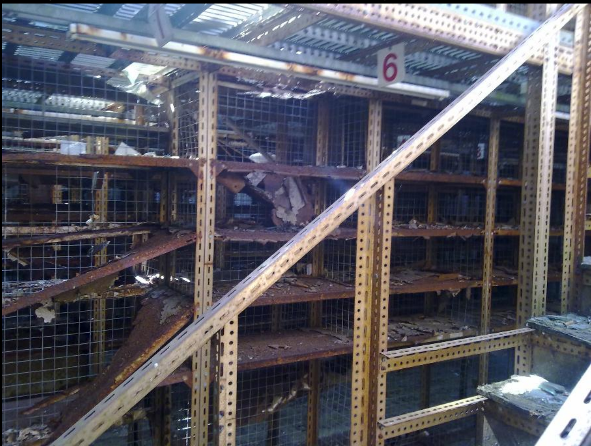
BELOW: The nut&bolt and fixings stores are something to behold. It must have taken several people quite a long time to construct this structure, as it is made entirely from pre-drilled angle iron. We aren't sure what sort of area this area covers, but it is sufficiently strong that walkways have been constructed over the top of it. Very impressive!
