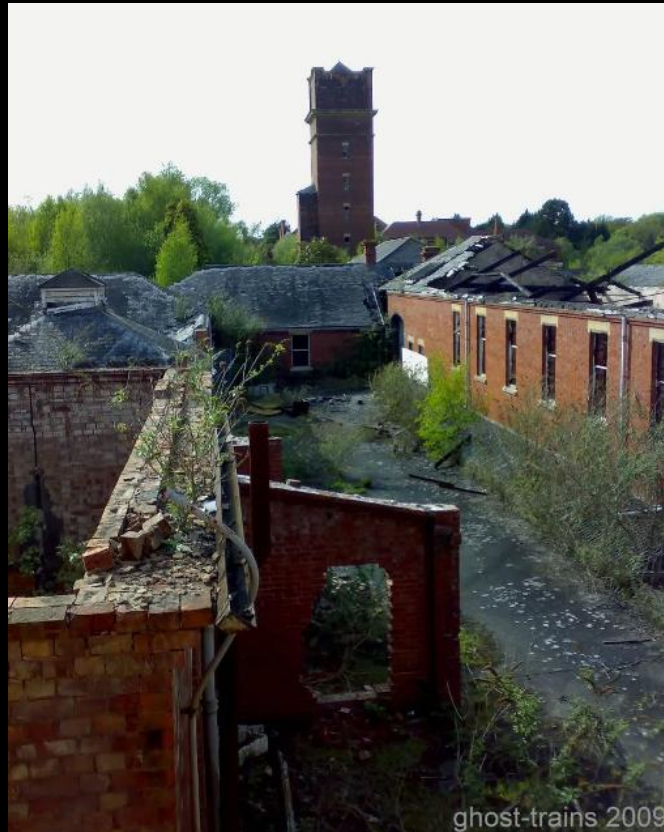
BELOW: Some brave residents battle on, despite the chaos of the demolition surrounding them.
