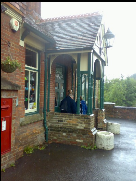
BELOW LEFT: It was about this point that it decided to piss down with rain, so we took shelter in the porte-clochere of the stationhouse and waited for it to ease off (and had a quick rollly as well).
