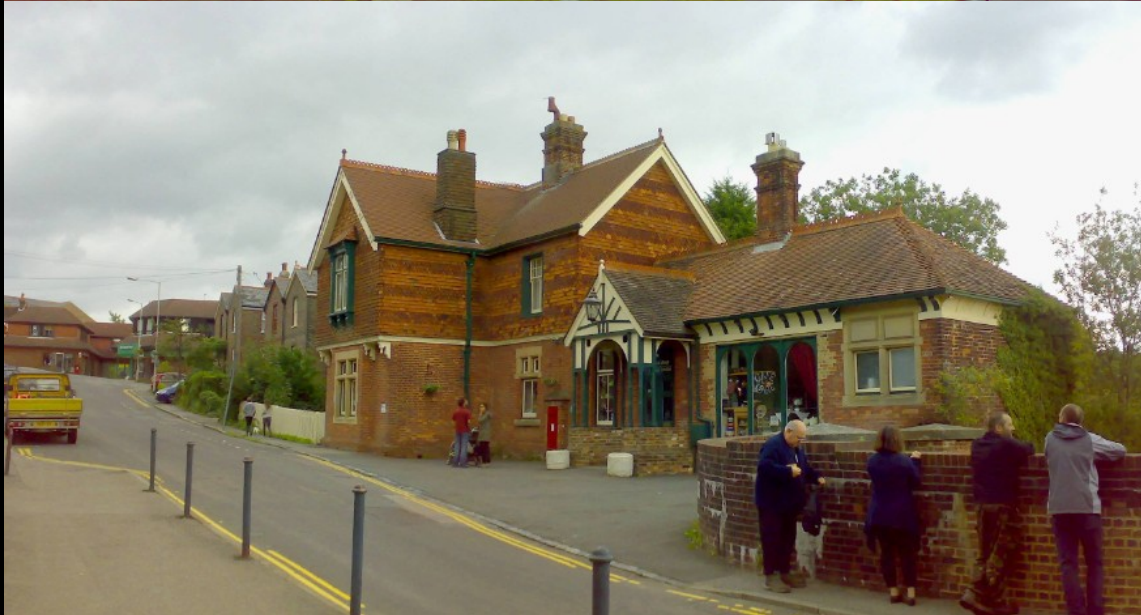
ABOVE: A nice 3/4 view of the station. The immediate area is relatively unchanged, but the inevitable ingress of newbuild modern tat is prevalent at the top of the road and stands out like a sore thumb.
