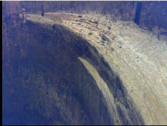
ABOVE: There are a few places along the tunnel's length where water drips through the ceiling and the ensuing limescale builds into the beginnings of stalactites.
