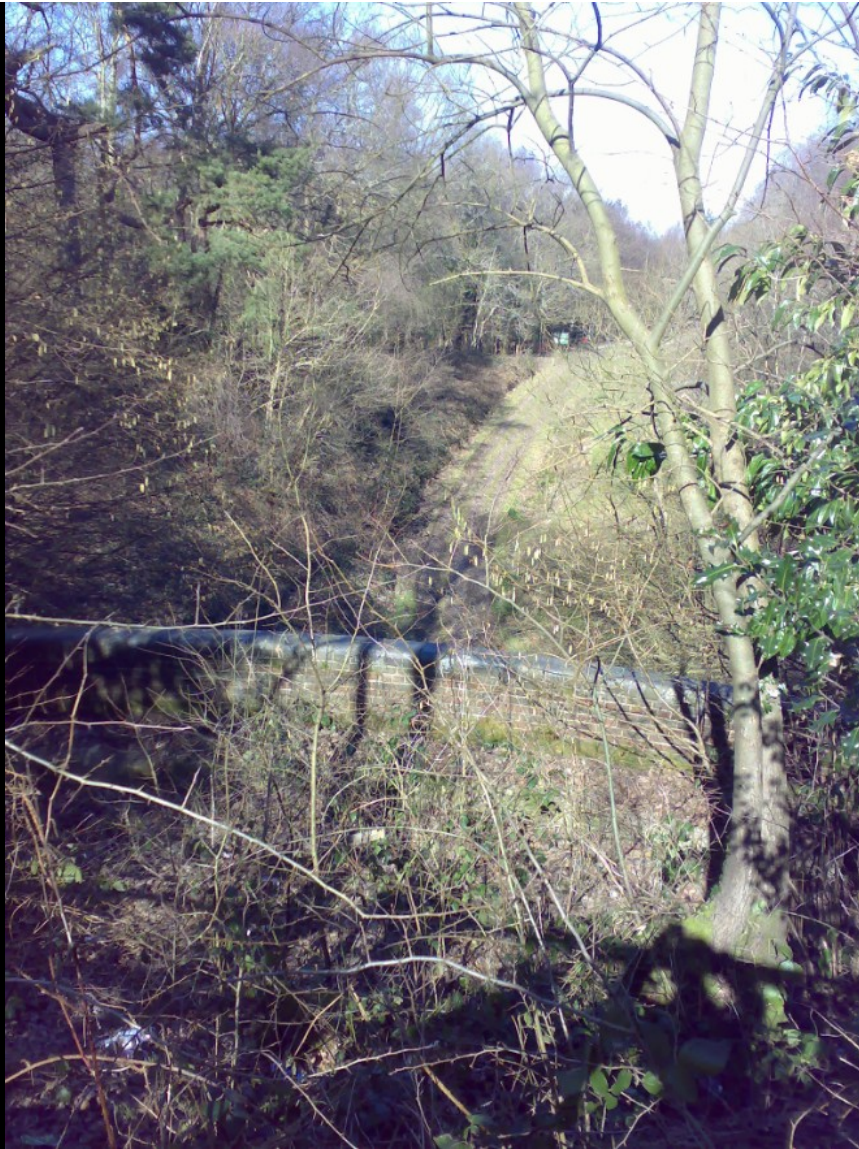
ABOVE: The trackbed, viewed from just above the parapet of the Heathfield Tunnel. The tunnel will be investigated in a lot more depth in a future trek, as it is open to the public during the summer season.
