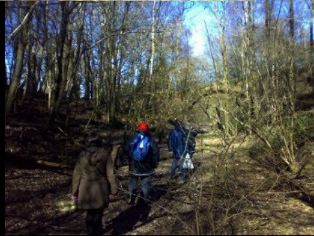
ABOVE & BELOW: This bridge carries a public footpath and access road to Colyton Farm over the trackbed. The area beyond is very private property, so we had to divert off the trackbed via the footpath at this point, otherwise we'd have had to cross someone's front garden and that's pushing it a bit far...
