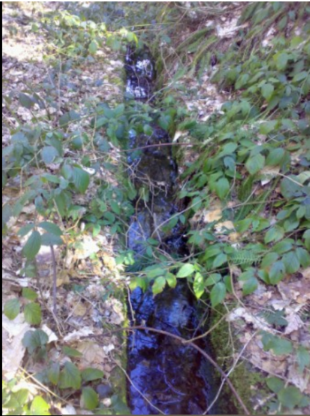
LEFT: At odd intervals along the trackbed, this little drainage channel would appear out of the scrub. It has obviously been cleaned out periodically, but even so, is in excellent condition considering.
