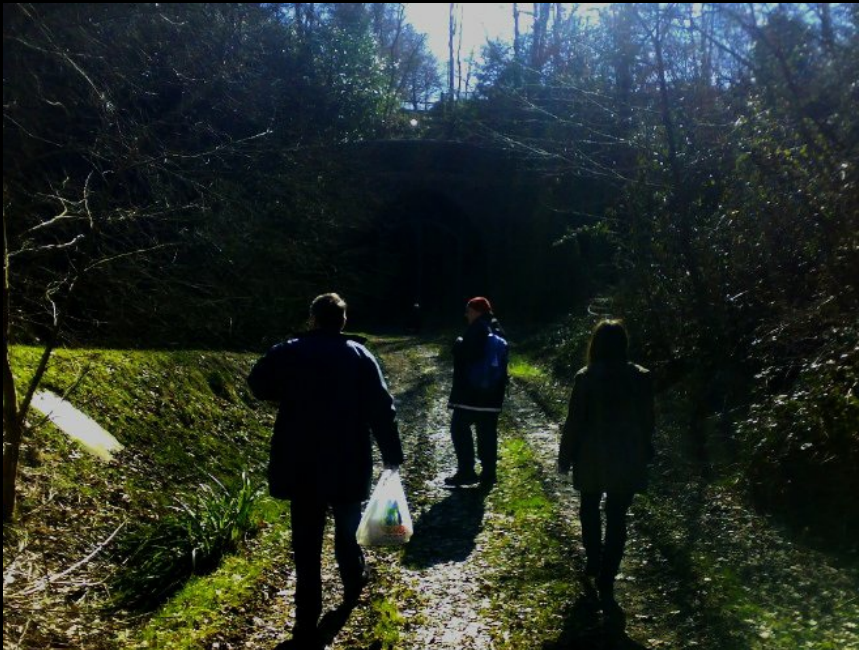
ABOVE: This is the start of the trackbed from the Northern entrance of the Heathfield Tunnel. The slope at this point is artificial and the original track level would have been a lot lower than this, otherwise the poor engines would have a considerable problem getting up here! Where the 3 Agents are standing, the track would have been approximately 5 foot lower.
