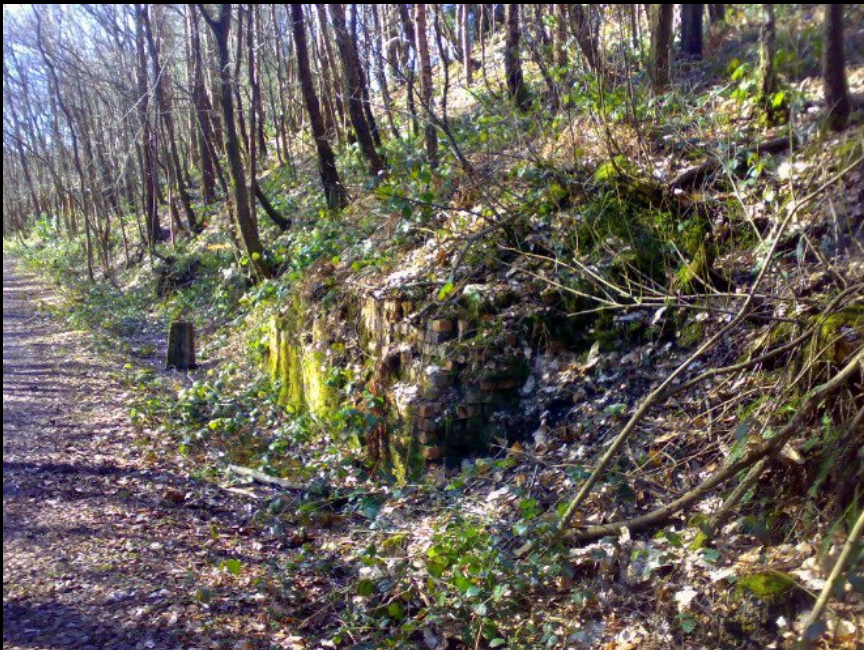
ABOVE: We are not too sure about this structure: at first we thought that it was the base of a grit bin platform, but on closer inspection, the brickwork has been very neatly faced up with aspects to north, south and east. It looks very substantially built as well, so more likely to be the remains of a small occupational bridge over the track. However, there is no corresponding pier on the opposite side of the cutting, so we are at a bit of a loss here.
