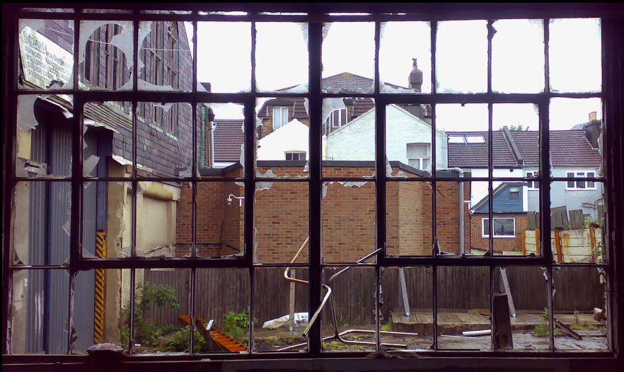
ABOVE: An arty window shot looking out from the ground floor of the warehouse. This view is looking due west. The back of Connaught House can be seen on the left.
