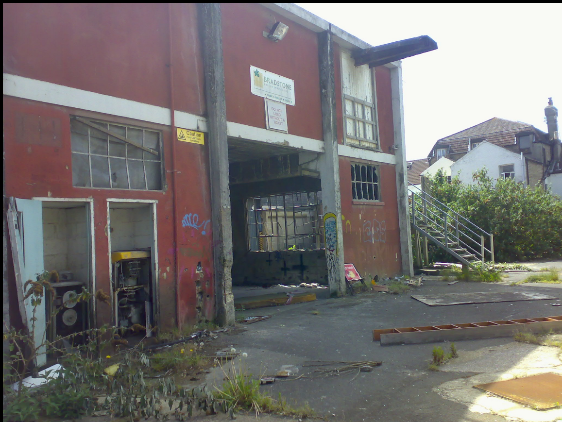
ABOVE: This warehouse type building is just to the left of the access gate and while there wasn't much in it that worthy of note, the stairs up to the top level allowed some good panoramic shots of the Hall, which is just round the corner of this building (to the left)
